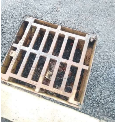
Blocked drain
