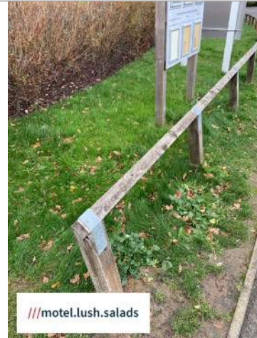
Acorn Park knee rail, posts are rotten, need replacing. Hunts Grove Drive
