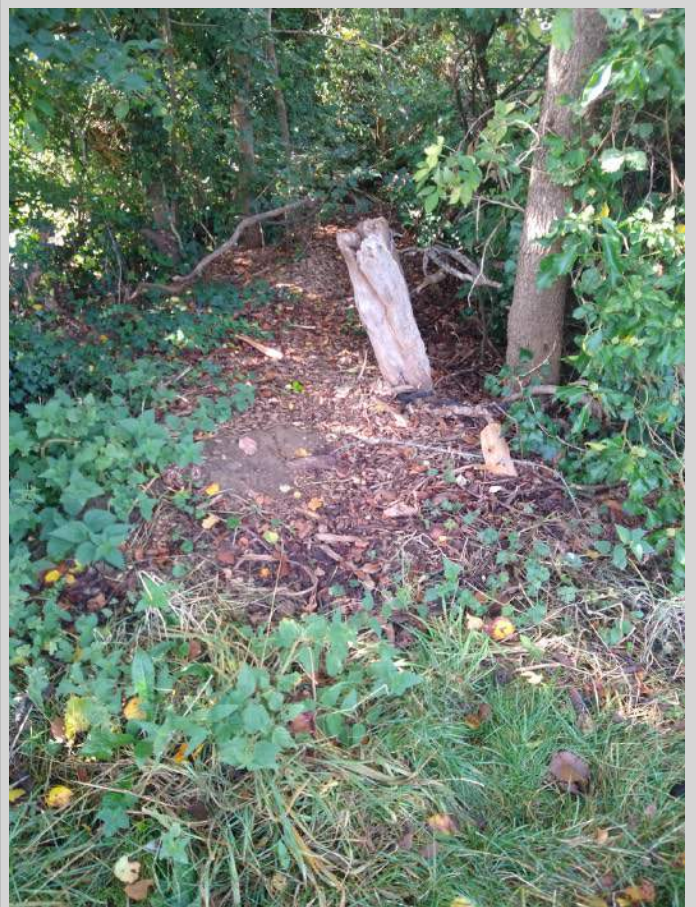
LUTRA CLOSE - Unmaintained hedgerows. Contains chippings dumped by Crest contractors as well as barbed wire that has been requested to be removed on a number of occasions.
