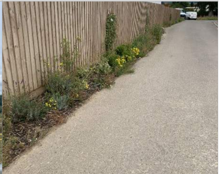
BOVIS - Weeds around site compound
