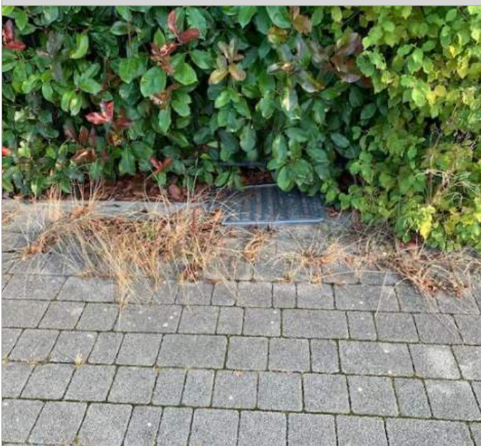
LIME TREE AVENUE - Weeds in pavement
