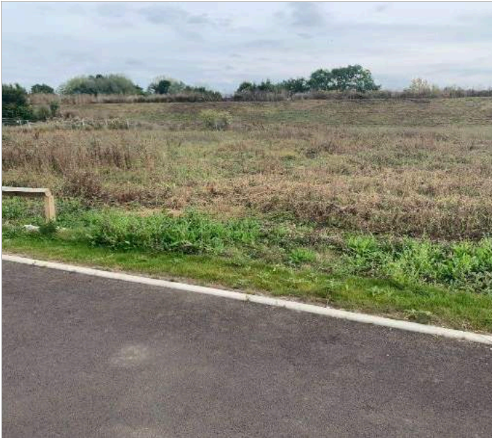
BELLWAY - Missing fence rails and overgrown with weeds
