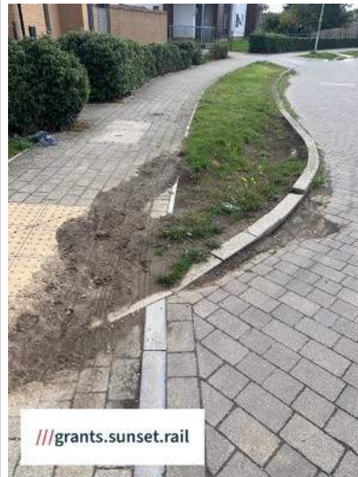
HUNTS GROVE DRIVE - collapsed kerbs
