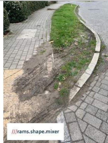
Damaged Verge Hunts Grove Drive
