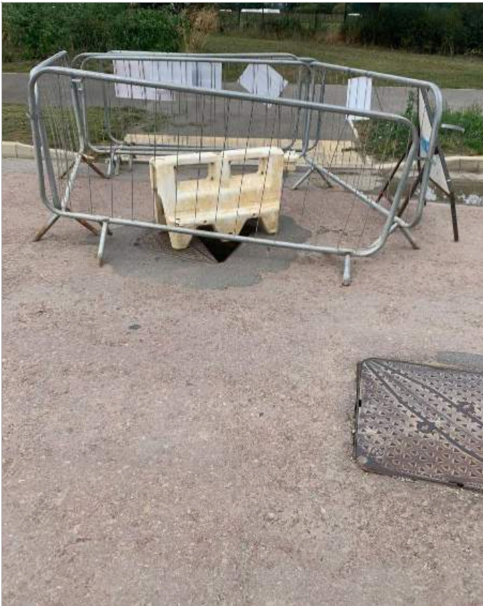
HARRIER WAY - Missing manhole cover
