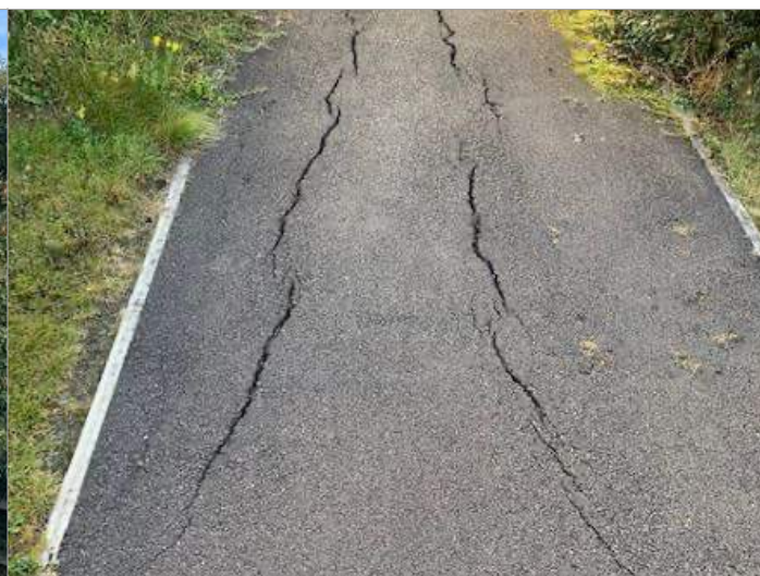
HUNTS GROVE DRIVE - Severe subsidence of path
