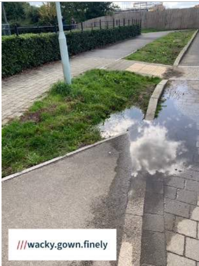
HUNTS GROVE DRIVE - collapsed kerbs and drainage issues
