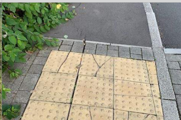
LIME TREE AVENUE - Pavers damaged
