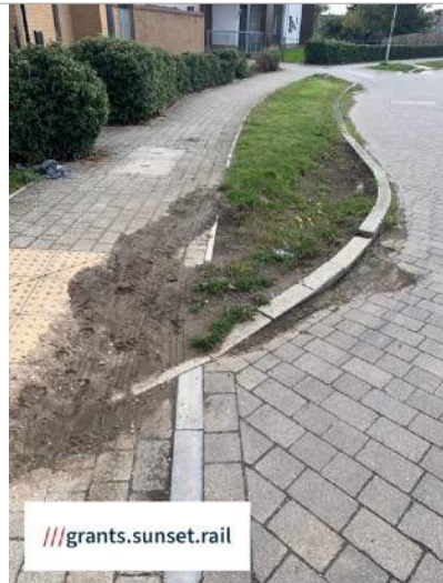
HUNTS GROVE DRIVE - collapsed kerbs
