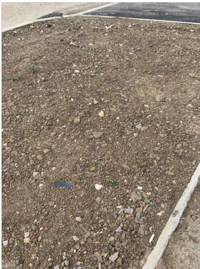
BOVIS - Poor quality of topsoil for verges
