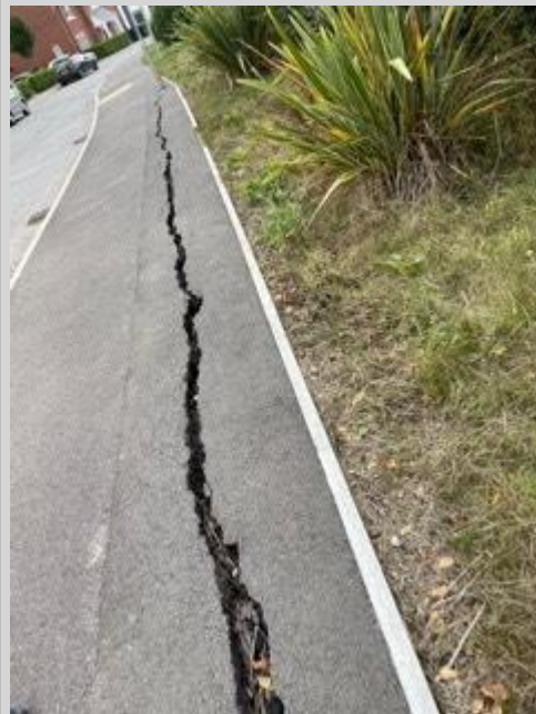
HARRIER WAY - Huge crack in tarmac leading to the bus stop.. photo references Harrier way 2 and 3
