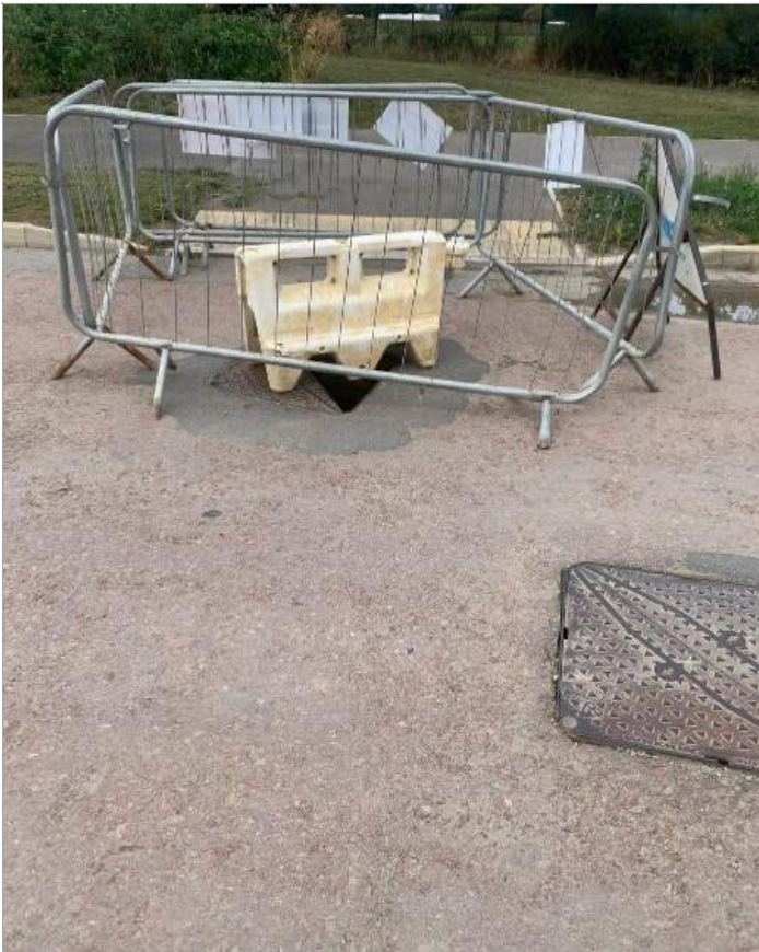
HARRIER WAY - Missing manhole cover
