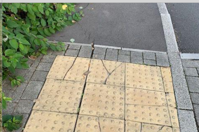
LIME TREE AVENUE - Pavers damaged
